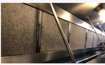
Woolguard hood filters capture 98% of airborne grease while still allowing air to pass through to the hood.
